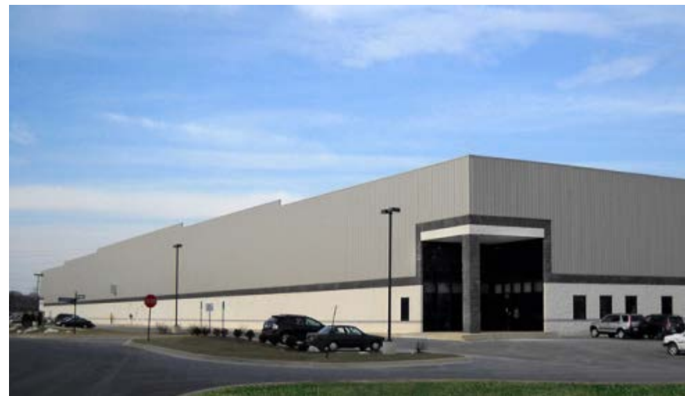
Twin Spans in New Castle
