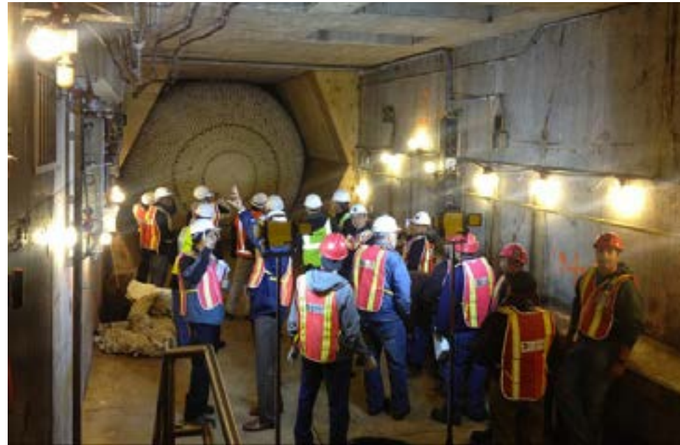
Officials in New York City take a look at ILC Dover's tunnel sealing technology in 2013.
